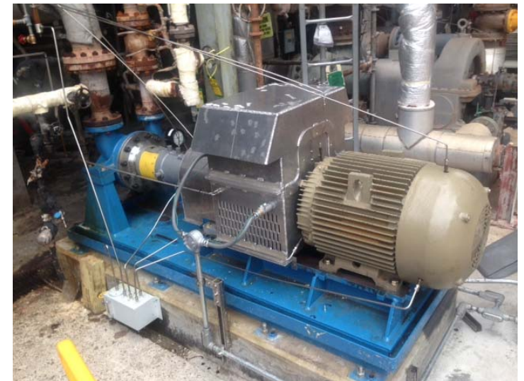
Picture courtesy of ExxonMobil in Baton Rouge, LA and MagnaDrive ASD solution
