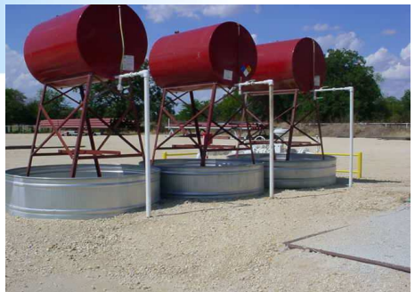
Day tank hoses replaced with sub-surface piping!
