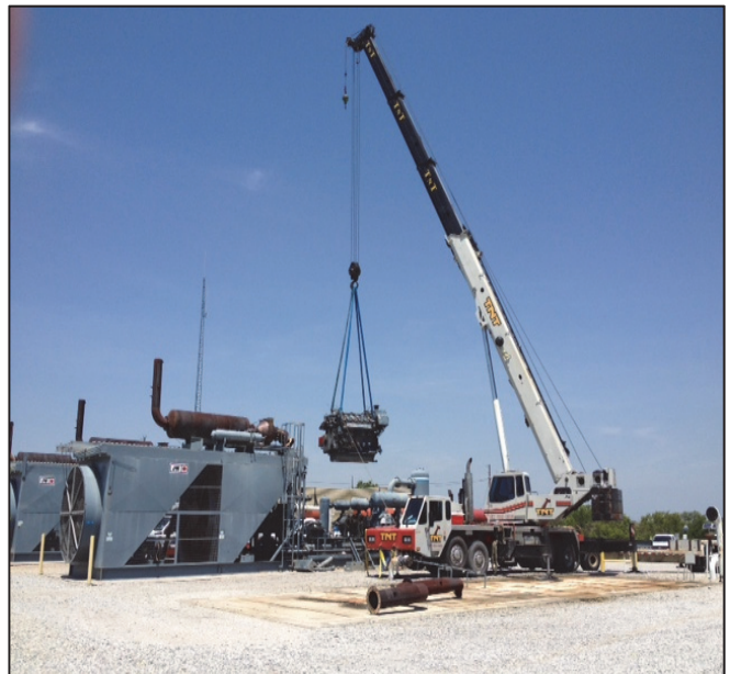
Figure 23: Larger horsepower packages generally require partial disassembly due to size and weight.
