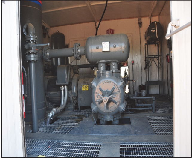
Figure 36: Enclosed packages must have space for performing routine maintenance.
