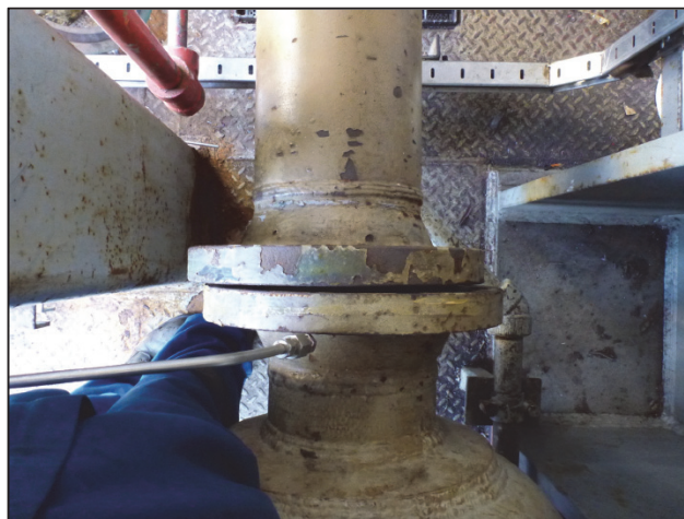
Figure 25: To avoid excessive strain, piping flanges must be well-aligned before assembly.
