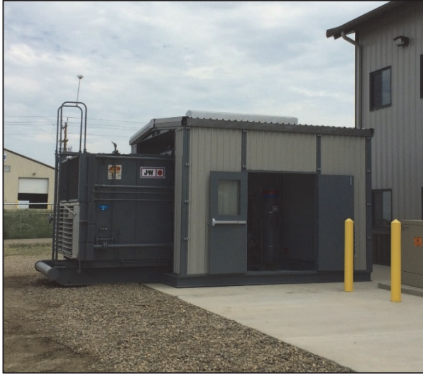
Figure 35: Consider an enclosed or Artic package for sites having ambients below 40°F.
