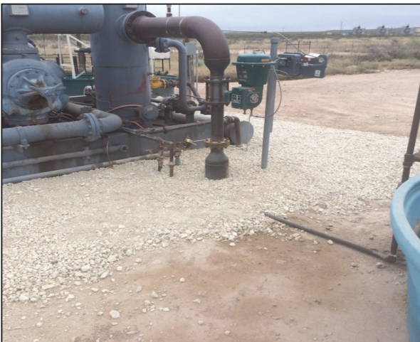
Figure 5: Gravel being installed to cover piping around a new compressor installation.
