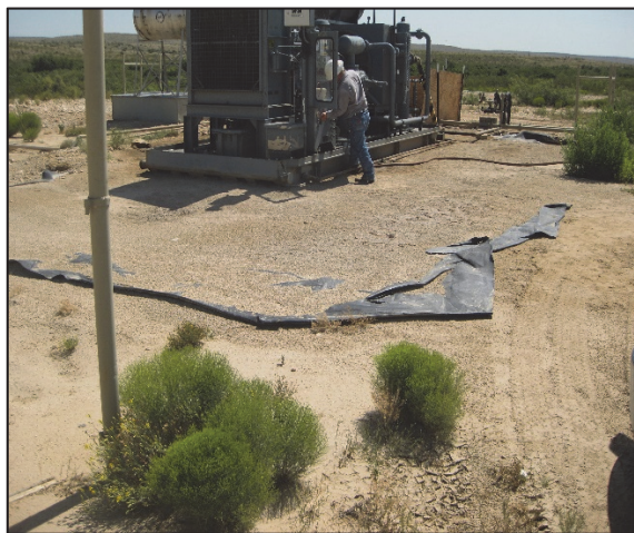
Figure 10: A layer of sand added over a plastic liner helps reduce slip/trip hazards.
