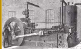
Straight-Line Reciprocating Steam Engine- Compressor
