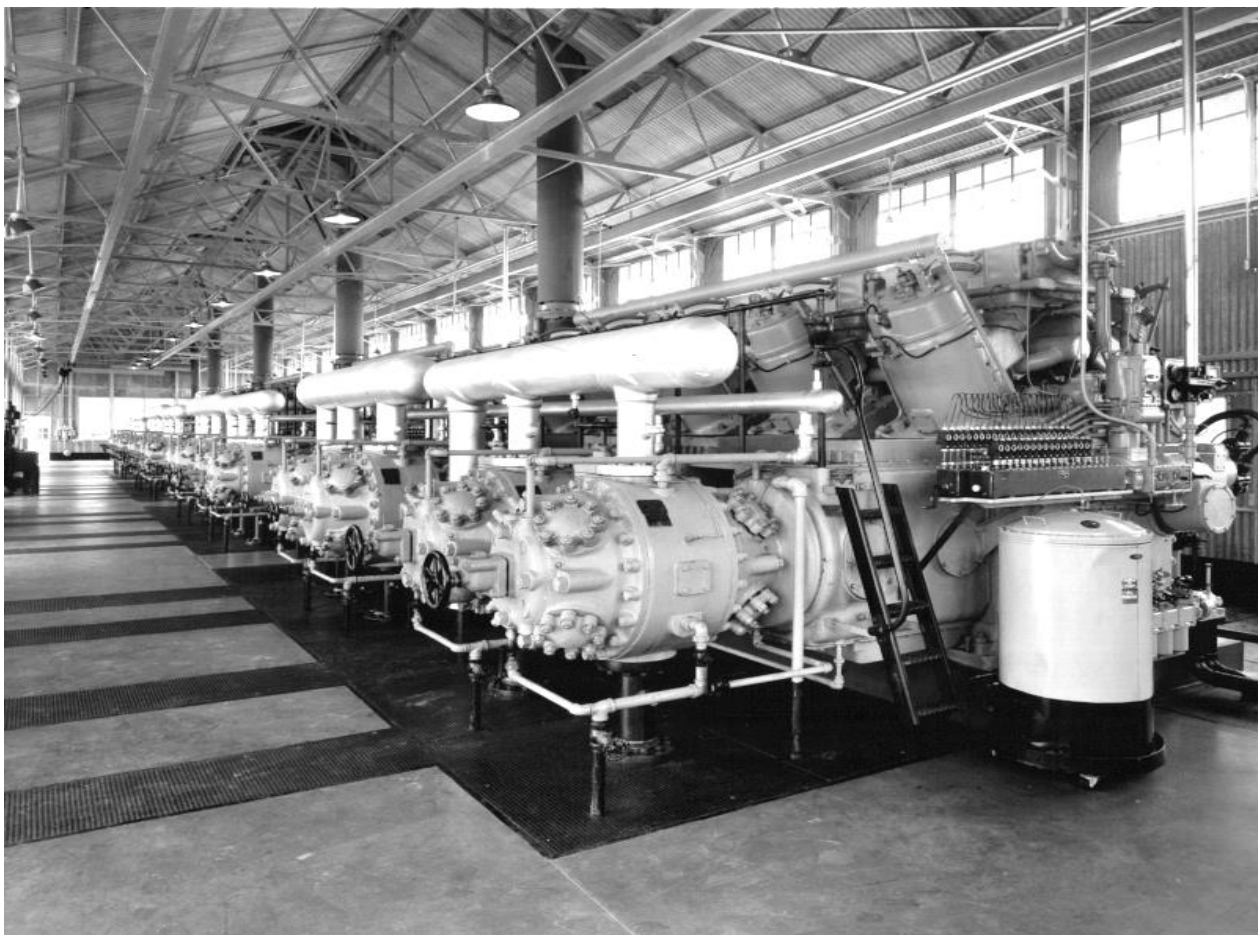
(6) C-B GMV-10 1950; C5 cylinder design originated in 1930s
